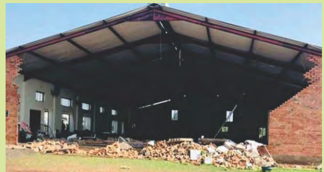
Figure 1: Images depicting (a) Radar imagery that depicts the storm that passed over the Empangeni, (b) image of the collapsed wall of the Pentecostal Holiness Church in the Empangeni area.
