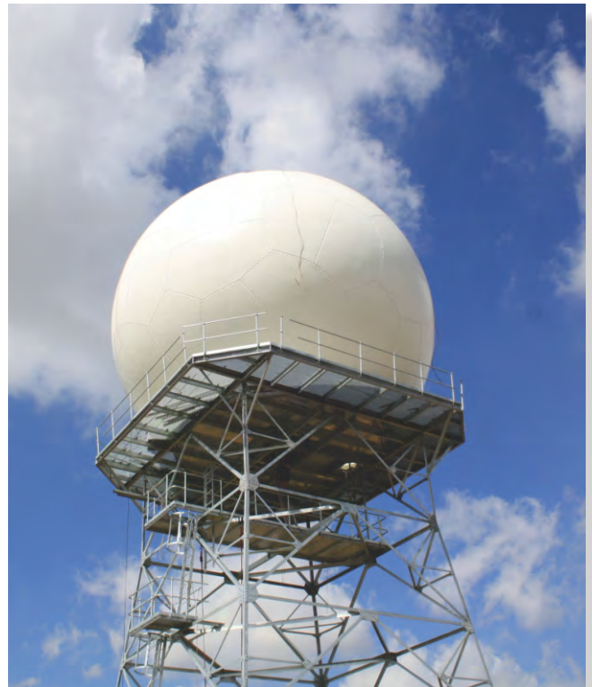
The Irene Radar is one of the ten S-band radars covering Gauteng, parts of Northwest, Mpumalanga, Limpopo and Free State with its coverage range of between 200 -300 km radius.
