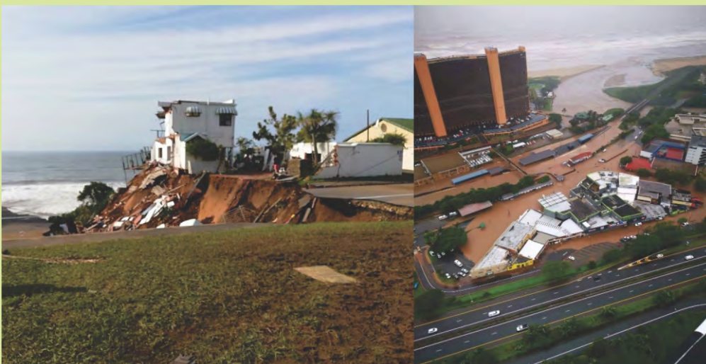
Figure 6: Collapsed house along the KZN coast and on the left an aerial view of flooded Amanzimtoti on 23 April (source: News24).
